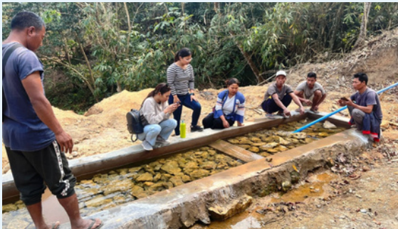
Inspection of OLC (Open Lime Channel) construction at Chima Dachit village.
