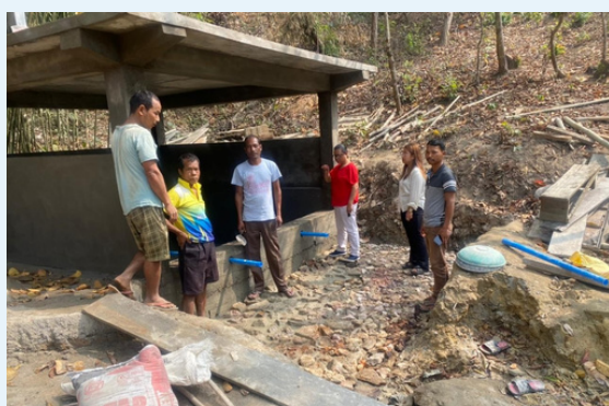
Site inspection on Spring Chamber (SRES) CATALYTIC FUND at Chiringpara village.
