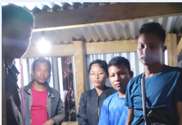
Successful installation of Hydroger at Paromgre Agro, Chokpot Block, South Garo Hills district.
