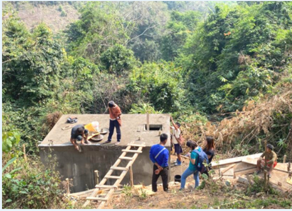
Inspection of constructed platform for water distribution and storage tank.
