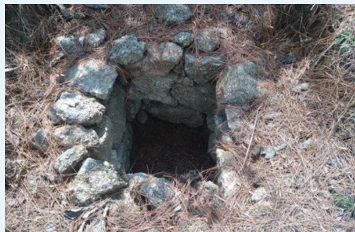
Inspection of recharge pit at Lai Kyntoit under Myllem Block
