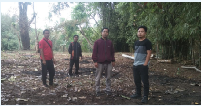
Site Visit to Gitokgre Village under Samanda Block, EGH, for Construction of Community Hall.
