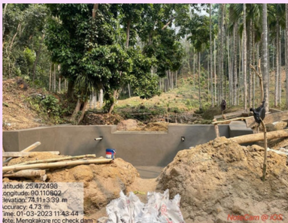
Inspection on RCC check dam Catalytic Fund by Field Engineer (EE)
