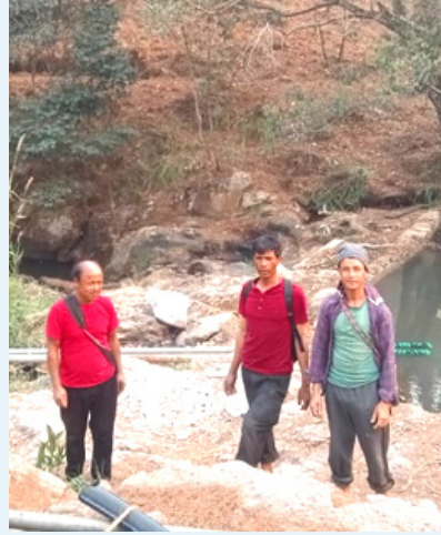
Inspection on installed hydro generator, On site operator training and testing and follow up on UC submission at Mynsngat village, Thadlaskein block West Jaintia Hills district.
