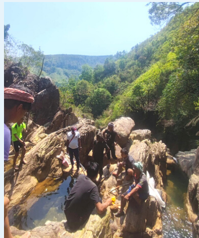
Site Visit for Electrification at Myllat Village, Pynursla Block, East Khasi Hills District.
