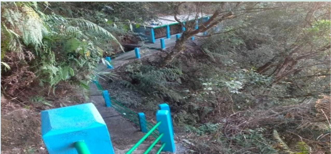
Fig: Phot Riat, spring chamber and safety rails
