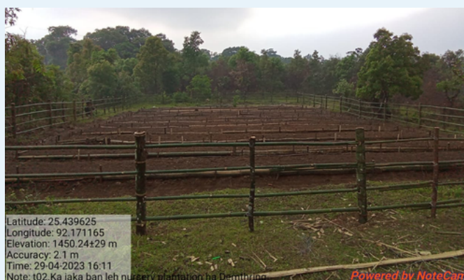
Work in progress at Demthring Village Nursery, Thadlaskein, WJH
