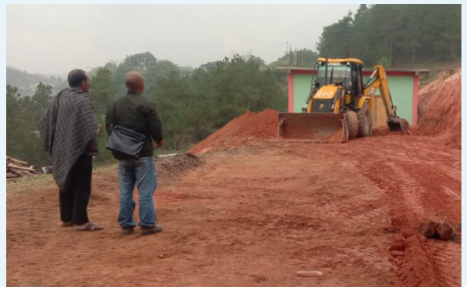
Earthwork at Sohtyngkhur Village, Mairang, WKH
