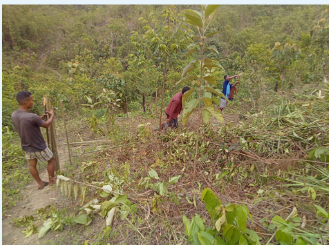
Stacking of poles at Dolwarigre Village, Samanda, EGH
