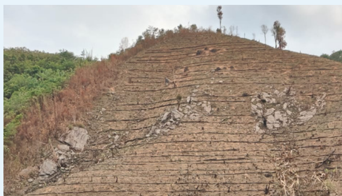
SALT farm prepared by Soil Department, EGH in Rongchekgre, Samanda Block, EGH.
