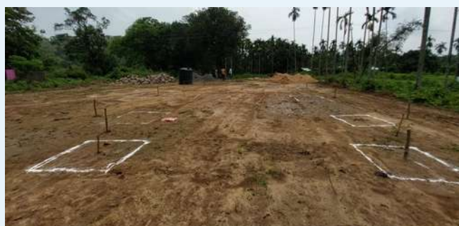
Footing Alignment, Rangdapara, Dalu Block
