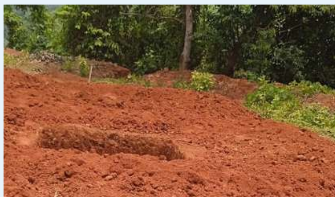
Excavation for footing in Simseng Rongal village
