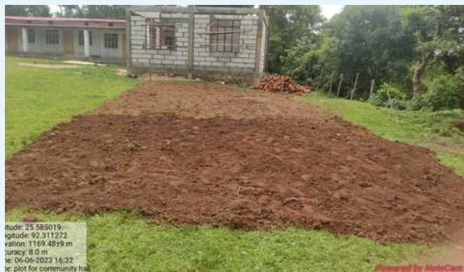
Work for Community Hall in progress at Madansynrang, Thadlaskein
