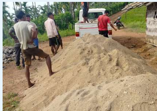
Boulders and sand delivered to Danal Dasik
