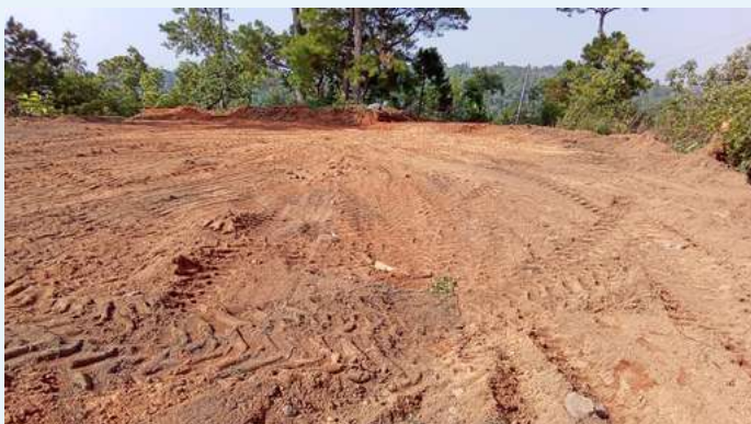
Work for Community Hall in progress at Iongsniehtakhniang, Thadlaskein
