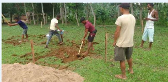
Ajasiram starting earthwork for Community Hall Construction
