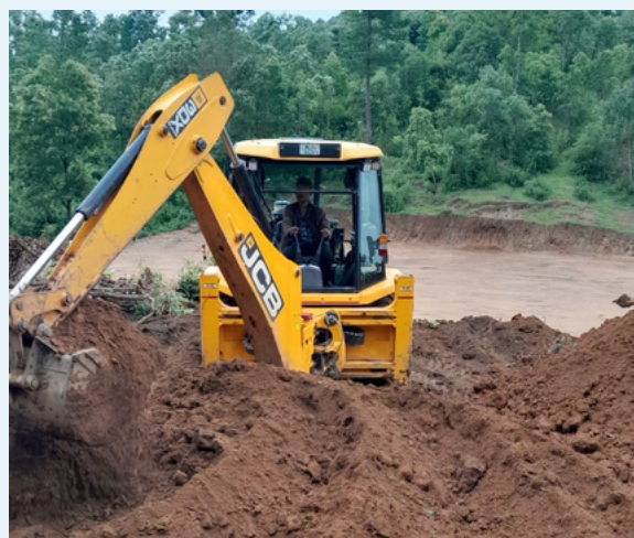
Progress of the community hall at Pdieniadaw village, Thadlaskein Block
