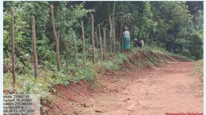
Fence poles have been erected in Derikgre
