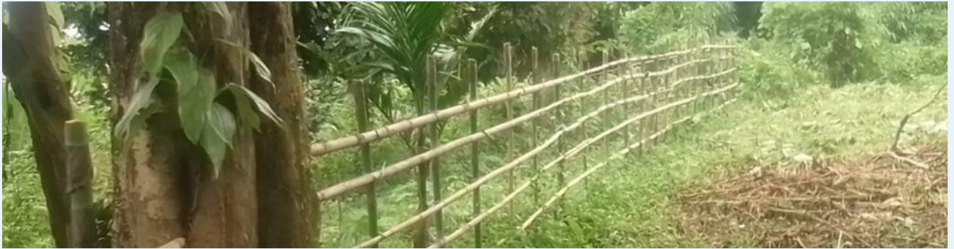
Fencing completed in Songmagiri village on August 11, 2023.
