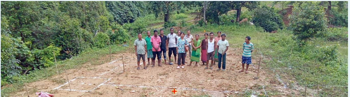
Aligning foundation for Bawagre community hall construction.
