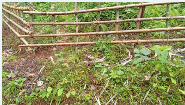
Fencing completed in Gambil Apal village.
