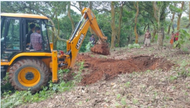
Earthwork at Adugre community hall.
