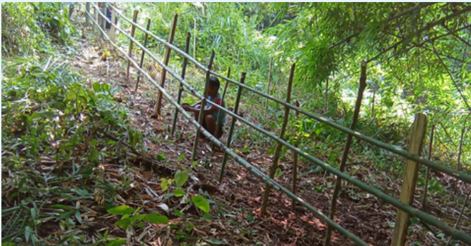
Fencing in progress in Dambo-Chare village.
