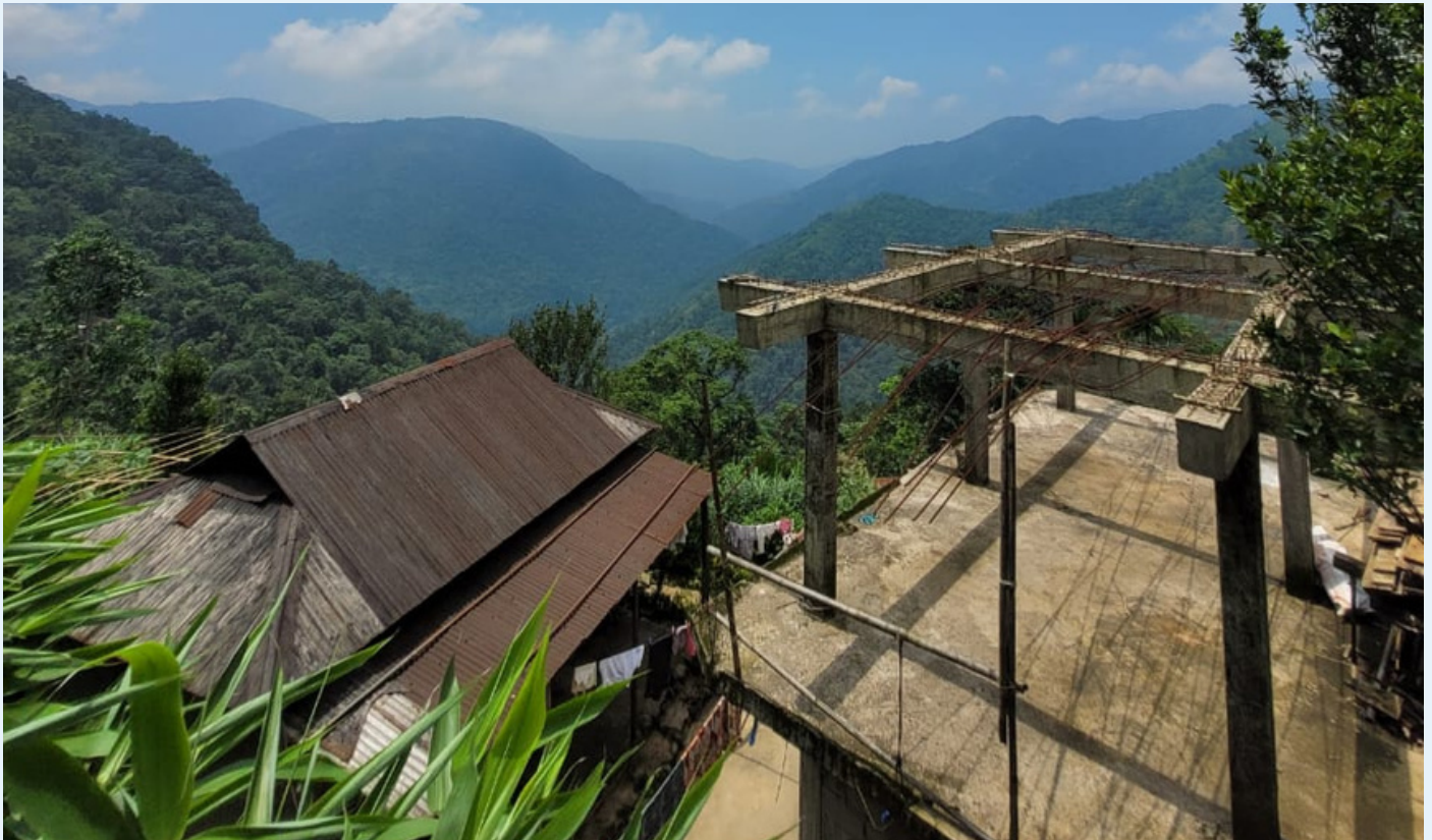
PES verification at Sarin village under Ranikor Block
