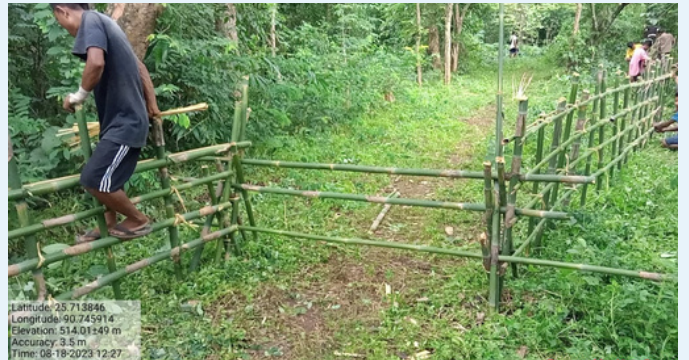
On August 18, 2023, the fencing task was completed in Rongchek Akong village.
