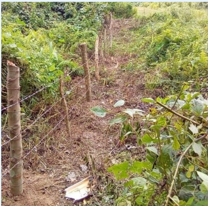
Fencing work at Anogre village.
