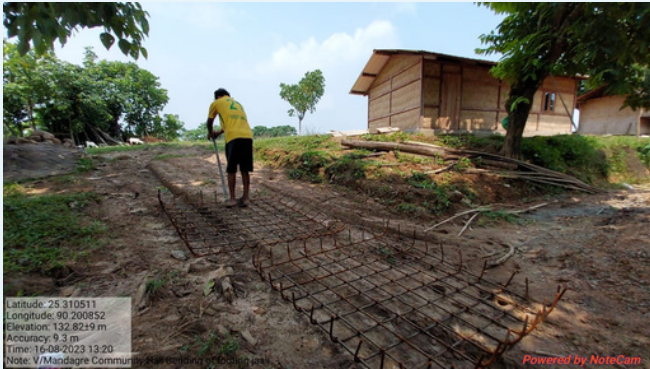
Elevation of footings and columns at Mandagre village.
