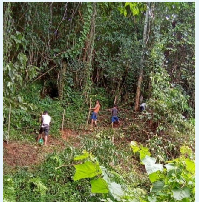
Fencing work at Renchagre village.
