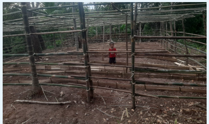
Nursery extension work at Attabengaon village.
