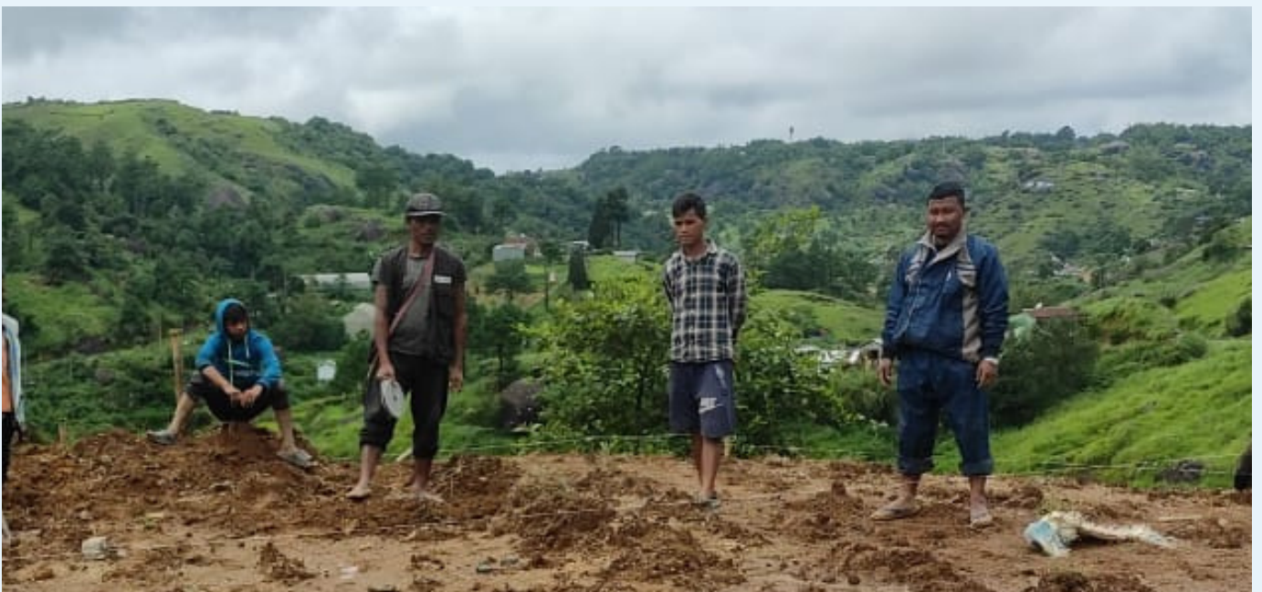
Alignment of column footing at Mawkyllung village.
